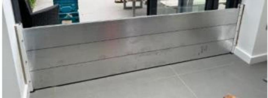
Above photos show an example of the works undertaken by our contractor. On the left is a non-return valve fitted to a waste pipe to prevent water backing up into the property. On the right is an aluminium slot in flood barrier to prevent surface water and fluvial (river) flows entering the rear of a property.
