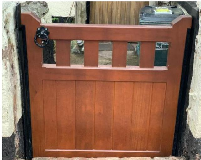
Photo of an installed flood gate in Stokeinteignhead
