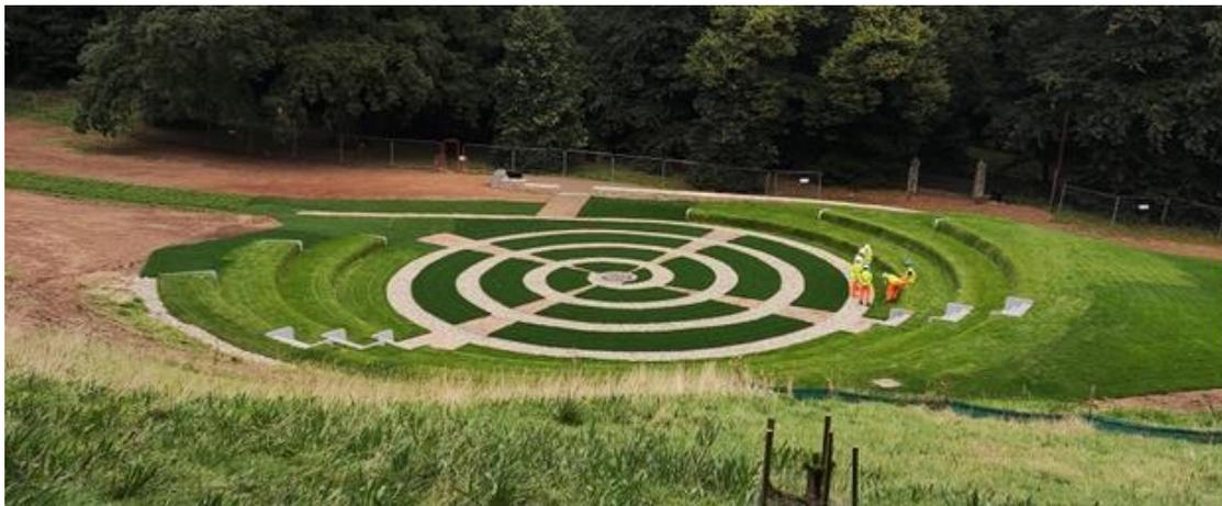
A key element of achieving planning permission for these essential flood attenuation scheme, was the requirement to make it a dual use space that could also be utilised as an amenity area for the local community when not in time of flood.
